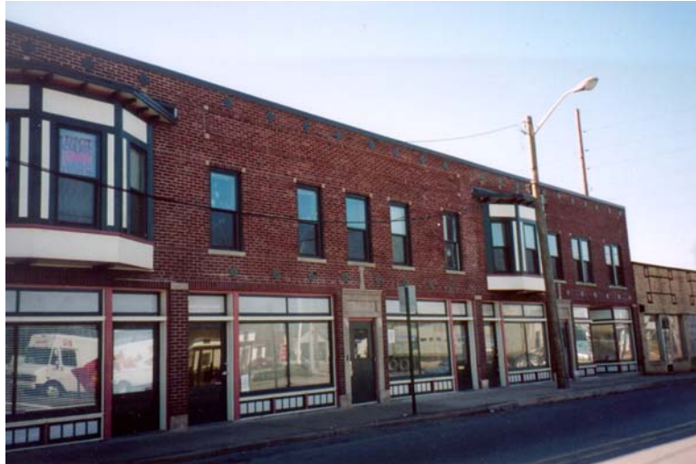
Located near the intersection of 10 th and Rural Streets, recently rehabilitated Mazingo Place (above) is one of several mixed-use buildings along East 10 th Street.
