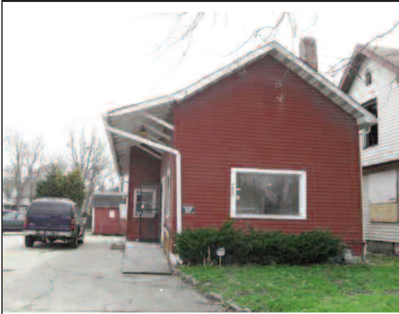
Front Facade as seen from East 10th Street
